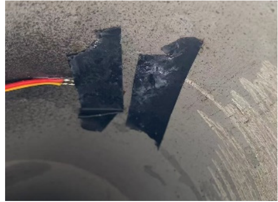
Fig. 5 Pasting of strain gauge inside the tunnel
