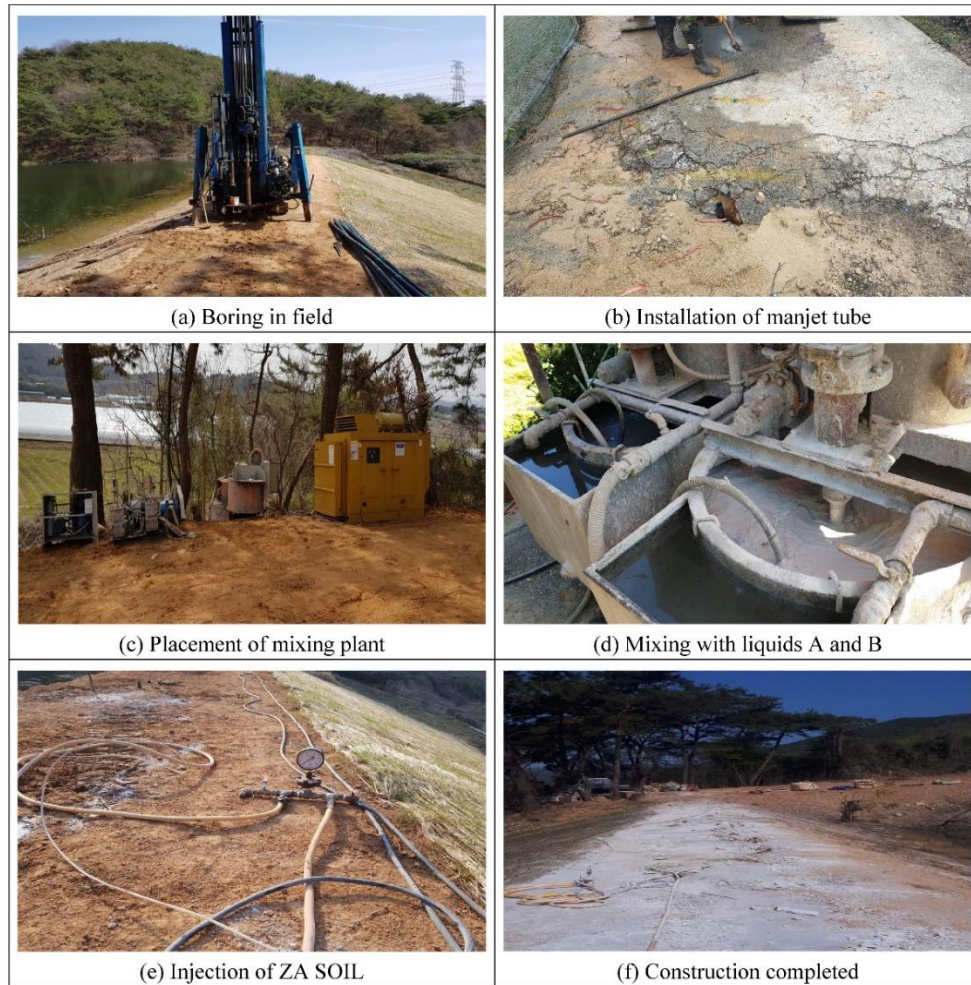
Fig. 6 On-site application of ZA-SOIL
