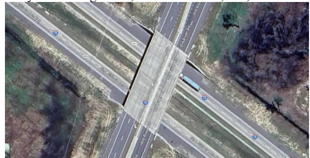
(b) Bridge 2-OR, at the intersection of I-16 and Old River Rd, near Meldrim, GA, USA
