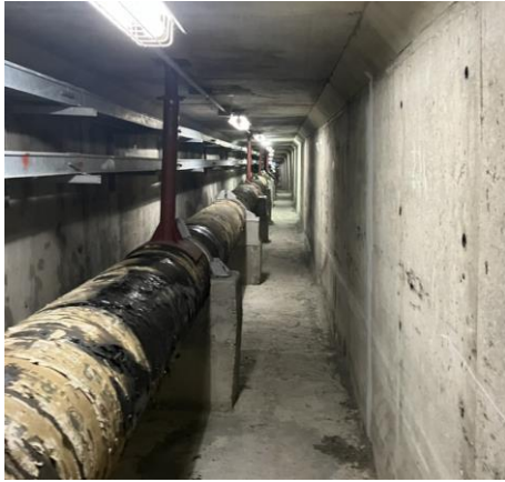
(a) Utility tunnel
