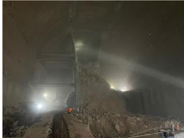
Fig. 1 Big tunnel section in the real site
