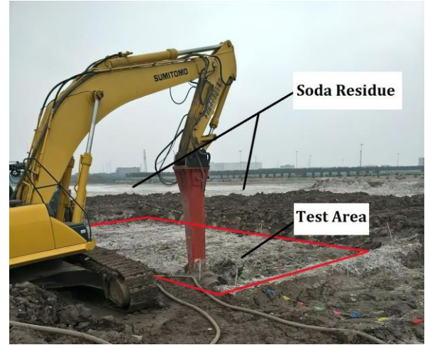
Fig. 1 In-situ stabilisation of soda residue
