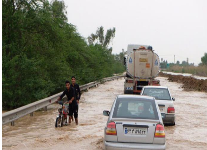
Fig. 1 A view of Ahvaz-Shush road after the flood in 2019
