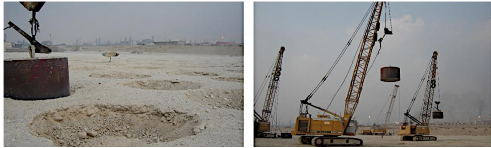
Fig. 7 Soil remediation of PSP by DC method
