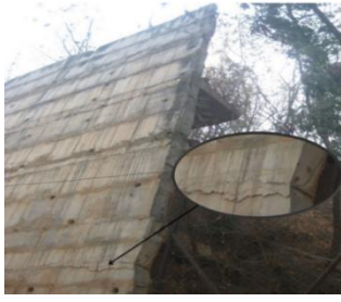
Fig. 1 Cantilever retaining wall with relief shelves
