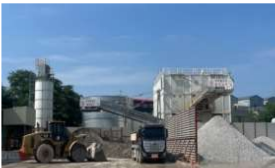
Fig. 2 Excavated materials after separation plant
