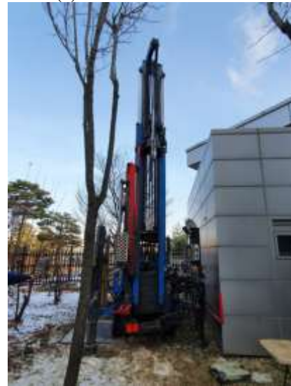
(b) Additional borehole drilling
