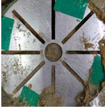
(b) Inside TBM chamber
