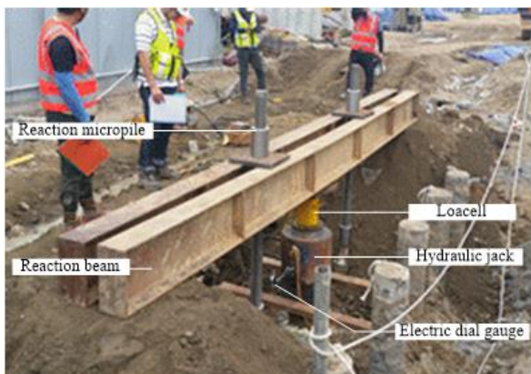
Fig. 5 Field compression test of micropile
