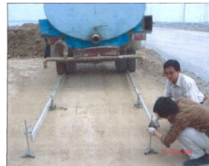
(c) Benkelman beam rebound deflection test
