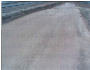
(a) Compacted expressway embankment
