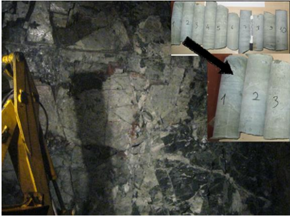
Fig. 9 Tunnel excavation face related to metabasalt and core samples
