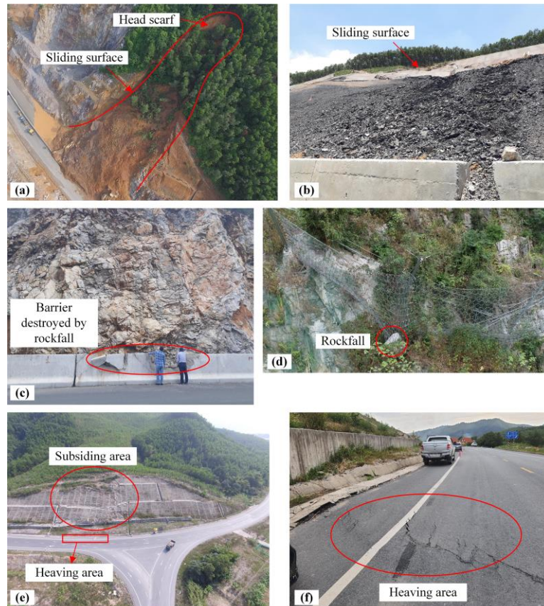
Fig. 2 Photograph of typical roadside landslides: (a) rotational slide at km 27+900; (b) translational slide at km 30+0.0; (c) rockfall at km 19+0.0; (d) and (e) spread at km 32+0.0
