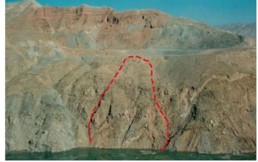
Fig. 3 No.2 landslide of Lijiaxia Hydropower Station
