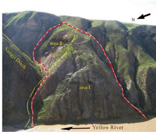
Fig. 4 No.3 landslide of Yellow River Hydropower Station
