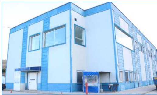
Fig. 15 EnerjiSA Üretim Bandırma-I NG CCPP, Control Building General View
