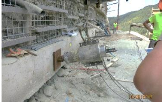
(a) Prestressing of anchors with a multi-jack
