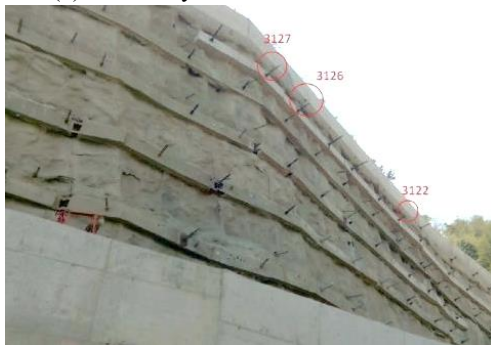
(b) View of one portion of reinforced slope
