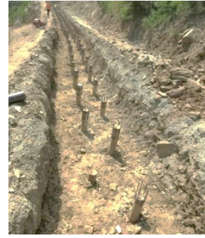
(b) Preparation works for connecting micropiles with capping beam
