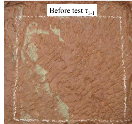
(f) rock mass surface before pouring concrete: natural weathering effect
