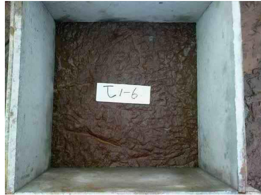
(b) rock mass surface before pouring concrete: no surface effect
