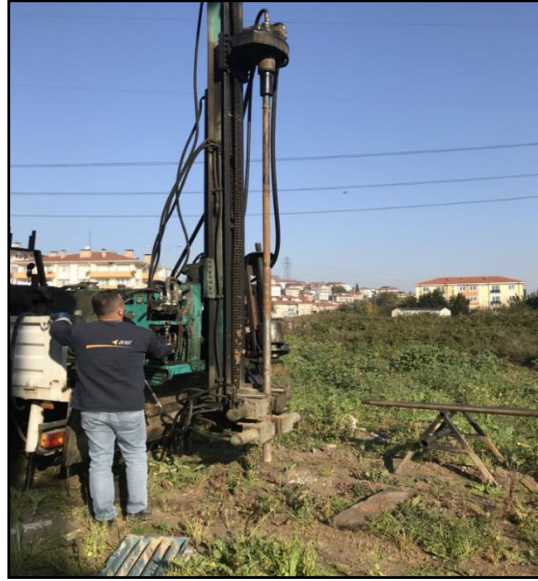
Fig. 5 Drilling work at the BH-1 point
