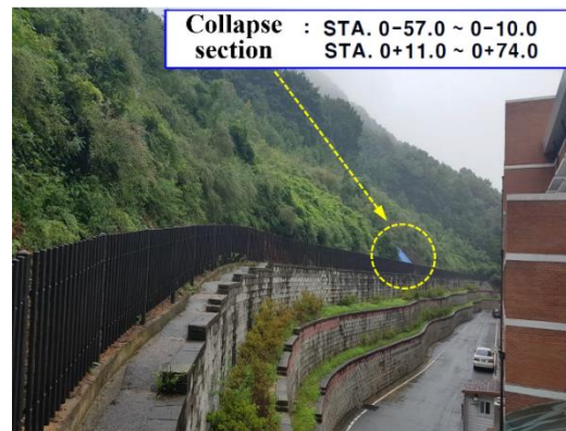
Fig. 4 Slope failure site behind the high school building
