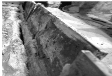
Fig. 6 Rotational failure for I-walls occurred for London Ave. Canal for test 2
