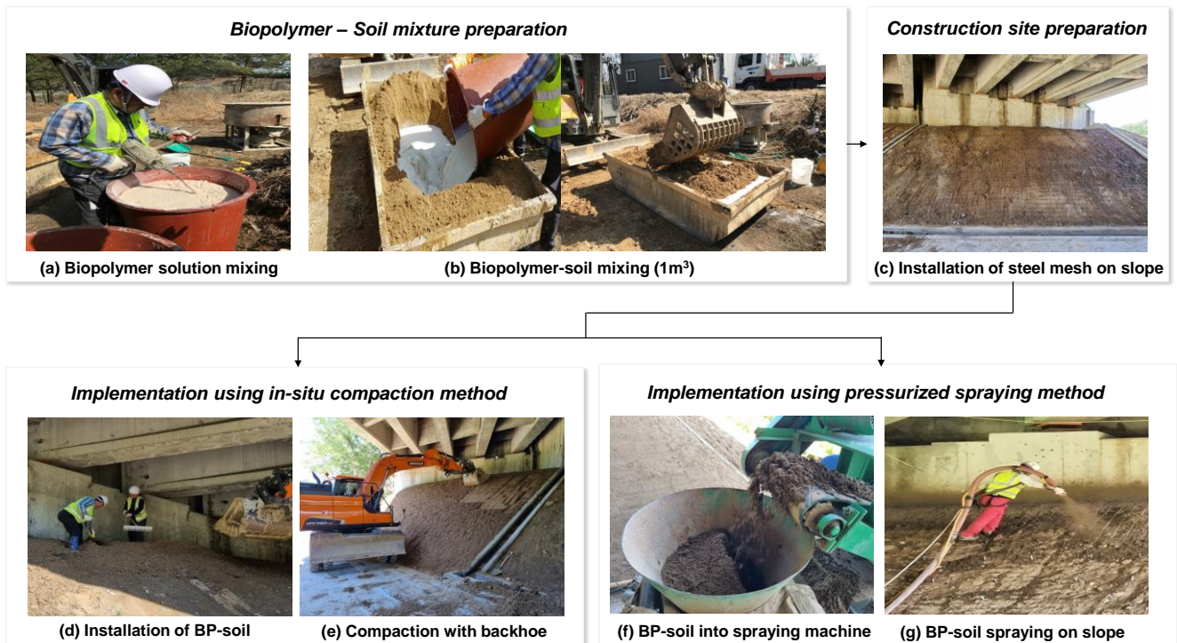
Fig. 4 Field implementation procedure of crosslinked biopolymer-treated soil
