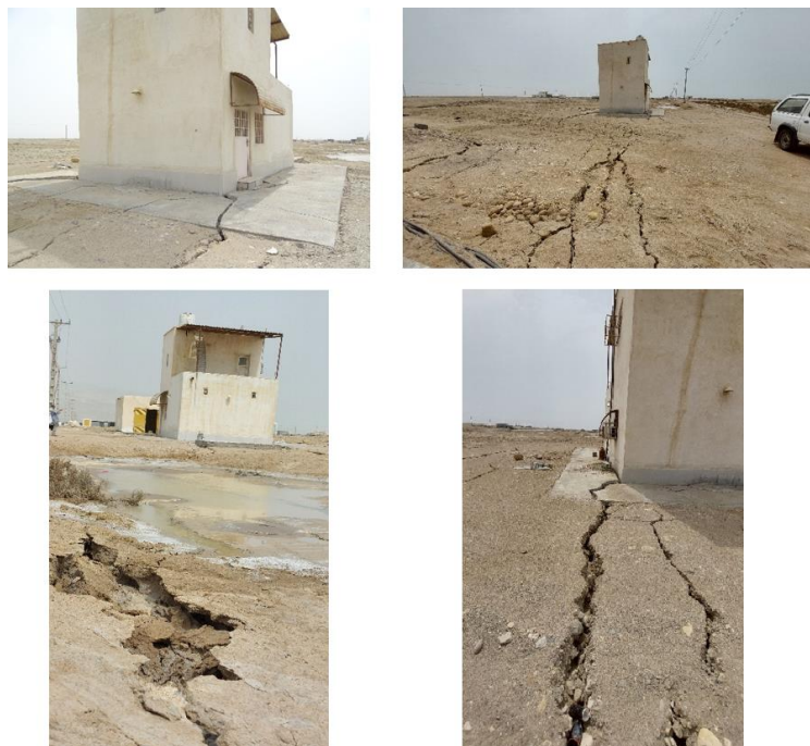
Fig. 28 A stiff building that tolerated nearly 20 cm settlement without considerable damage
