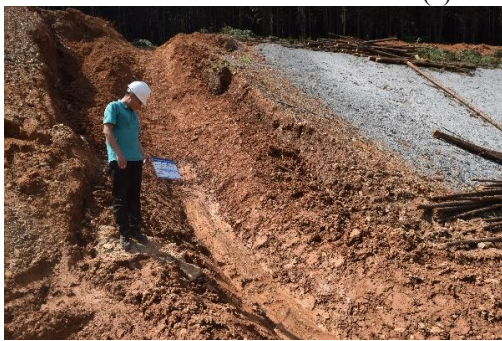
(b) Water inflow area
