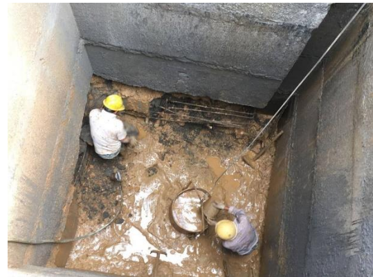
(b) Excavation of anchor piles
