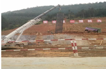
(c) Addition of anchor piles
