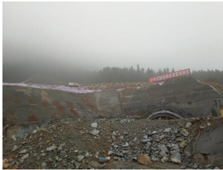
(a) Earth and rock backfill
