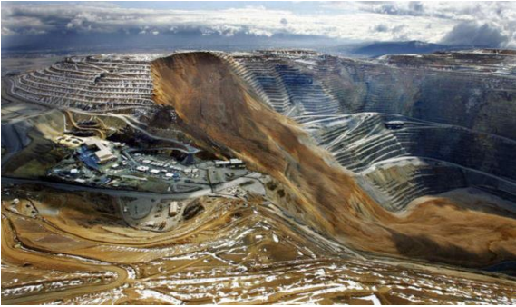
Fig. 1 A massive slope failure occurred at the open pit of the Bingham Canyon Mine in Utah (Kolapo et al. 2022)
