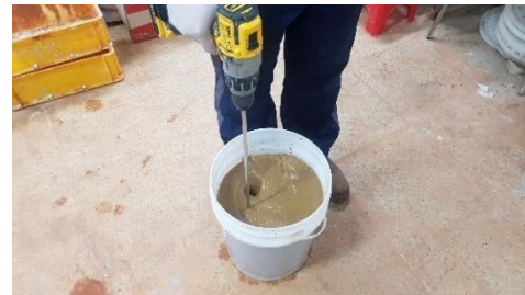
(b) Mixing process of bentonite slurry for 2 min.
