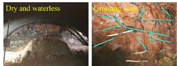
(b) Advanced grouting effect
