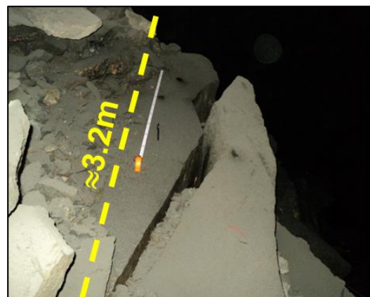
(b) Fallen rock from the back of stope at a depth of 693 m between two post-pillar at a distance approximately 20 m
