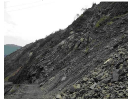
Fig. 2 Schematic of buckling slope failure and example of slope undergoing buckling failure in southwestern (Qi et al. 2015)
