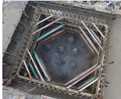
(c) Overview of constructed USSP cofferdam
