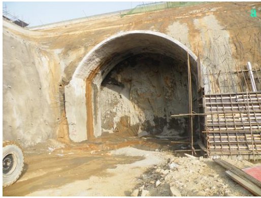
(a) initial segment of construction tunnel ①
