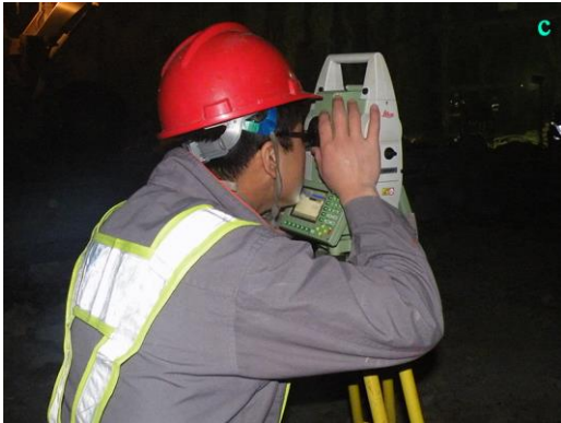
(c) settlement measurement using a total station
