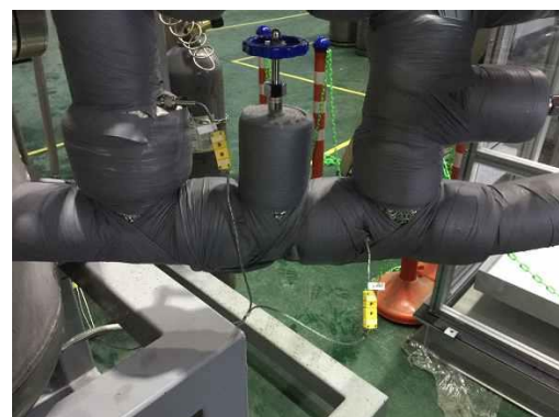
(b) Insulated bypass pipes
