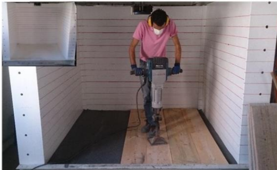
Fig. 2 Preparation of the first layer of sand bed with a relative density of 65% and vibratory compaction shown on top of wood pieces
