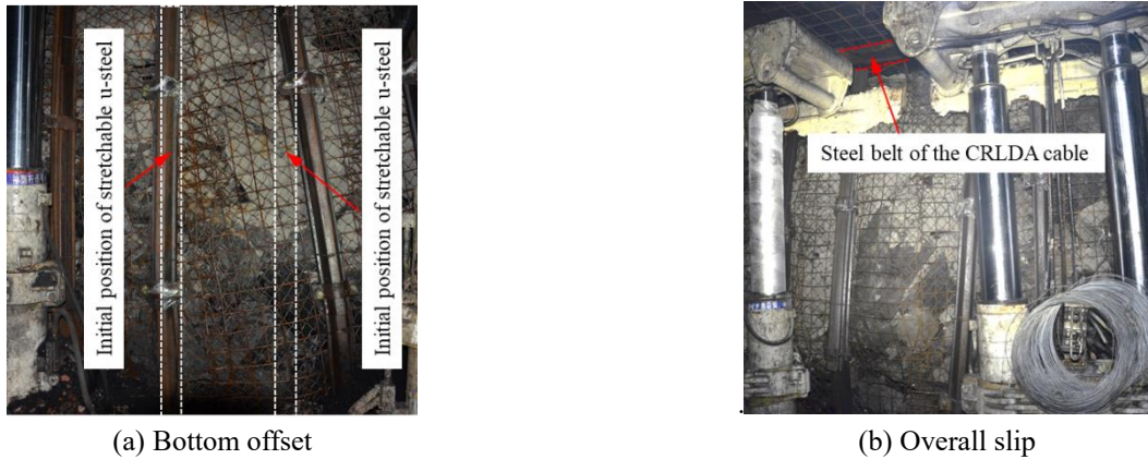
Fig. 15 Deformation types of the gangue support structure at the gangue side
