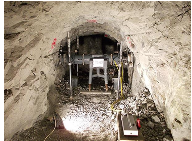
Fig. 2 Actual photo taken during the plate loading testing at Yusufeli Dam site (DSI 2015)
