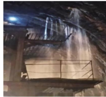
Fig. 11 Water inrush diagram of construction site (Xian et al. 2019)
