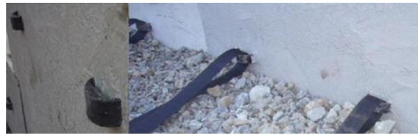
(b) Close view of drainage layer
