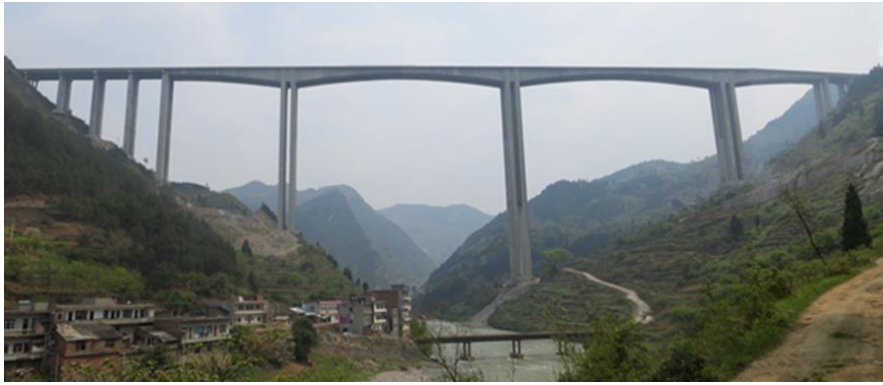
Fig. 1 Photograph of Tongzi River Bridge
