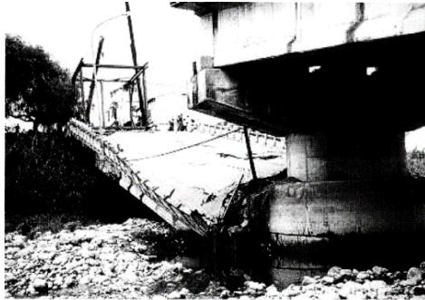
(a) Beam falling of the Xin-Yi Bridge
