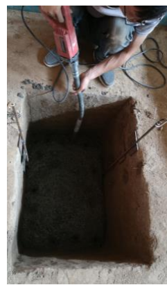
(c) Concrete pouring
