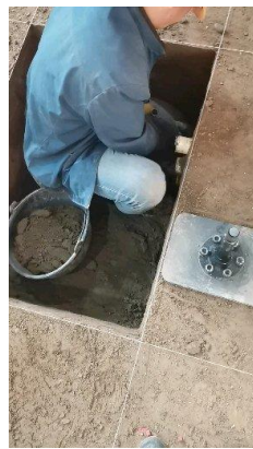
(b) Foundation pit excavating
