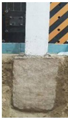
(a) Foundation of D-1
