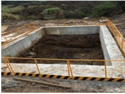
Fig. 1 Digging well foundation of HST high-speed railway bridge
