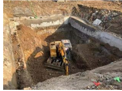
Fig. 1 Digging well foundation of HST high-speed railway bridge
