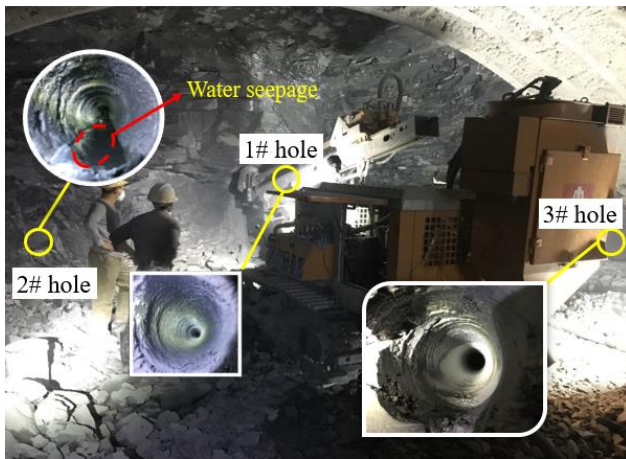
Fig. 6 Advanced horizontal drilling and groundwater condition
