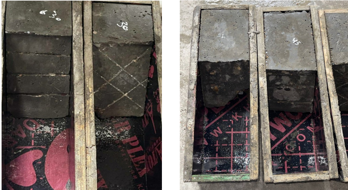
Fig. 13 Prepare surface plastic concrete prism beam
