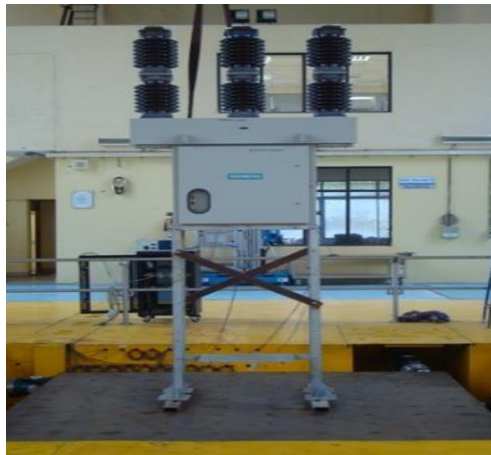
Figure 3. 36 kV circuit breaker mounted on shake table
