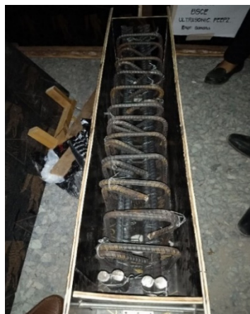
Fig. 1 Deformed Reinforcement Bar inside the beam mold
