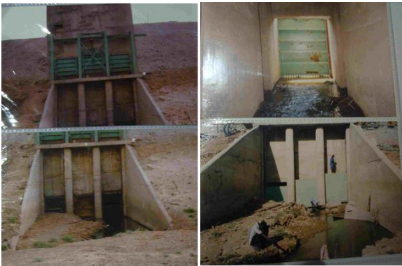
Fig. 18 Sluice gate of upper upstream gate dam 1
