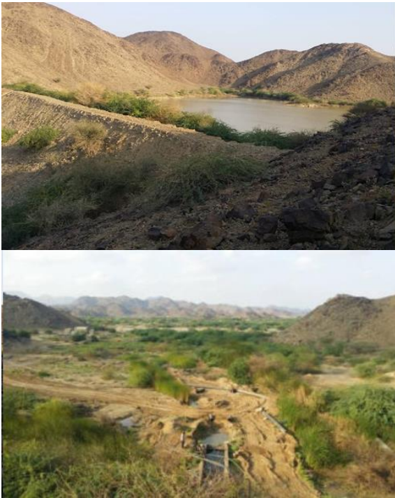
Fig. 20 Fourth reservoir embankment and intake
