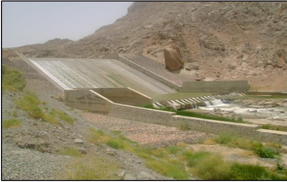
Fig. 17 Sluice gate and spillway of upper gate dam 1
