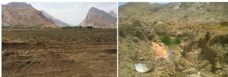
Fig. 33 SPC dam 2 before removal and dry siltation on SPC reservoir, 2019
