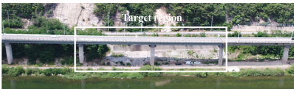
Fig. 1 Target region of the bridge
