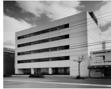
Fig. 1 The Kajima-Shizuoka Building
