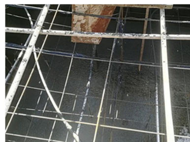
(b) Construction process
