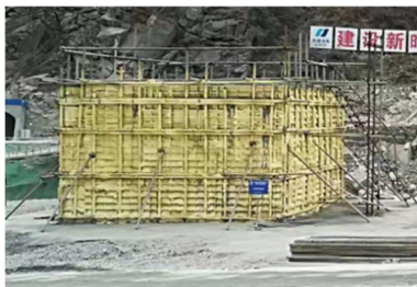
(c) Spraying of insulation materials before demolding
