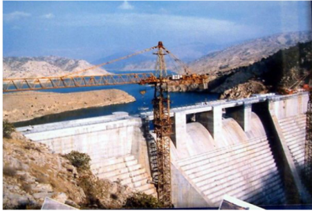
Fig. 1 Stepped spillway of Kosar dam (2006)
